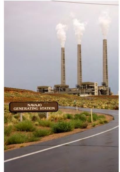
The Navajo Generation Station (NGS) consists of three coal-fired supercritical steam electric generating units with a total net capacity rating of 2,250 megawatts (MW). Unit 1 began commercial operation in 1974; Units 2 and 3 followed in 1975 and 1976. SRP is the plant operator.
