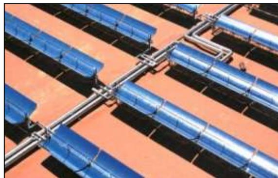
**Figure 6: (Top) Parabolic concentrator optical diagram. (Bottom) Solargenix SGX-1 solar collector troughs at SEGS site (source: Solargenix). Collectors usually track the Sun from East to West rotating about a North-South axis.**
