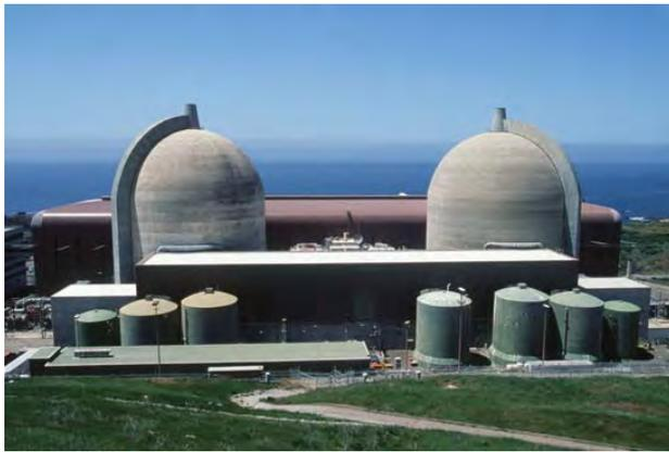
The most common nuclear power plant design uses a Pressurized Water Reactor (PWR). Water is used as both neutron moderator and reactor coolant. That water is kept separate from the water used to generate steam and drive the turbine. In essence there are three water systems: one for converting the nuclear heat to steam and cooling the reactor; one for the steam system to spin the turbine; and one to convert the turbine steam back into water.
